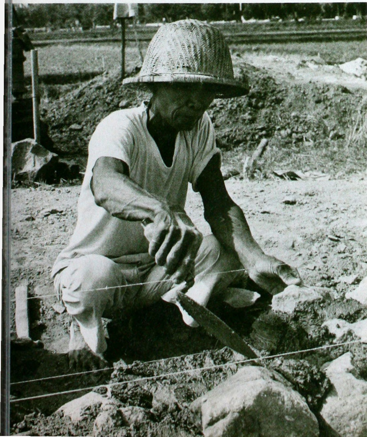
The first stage of construction of an orphanage that will house 100 children in Pare, Indonesia
