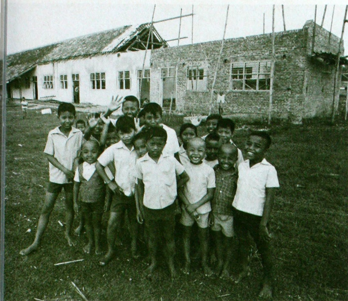
Children in front of a new addition being built for their school
